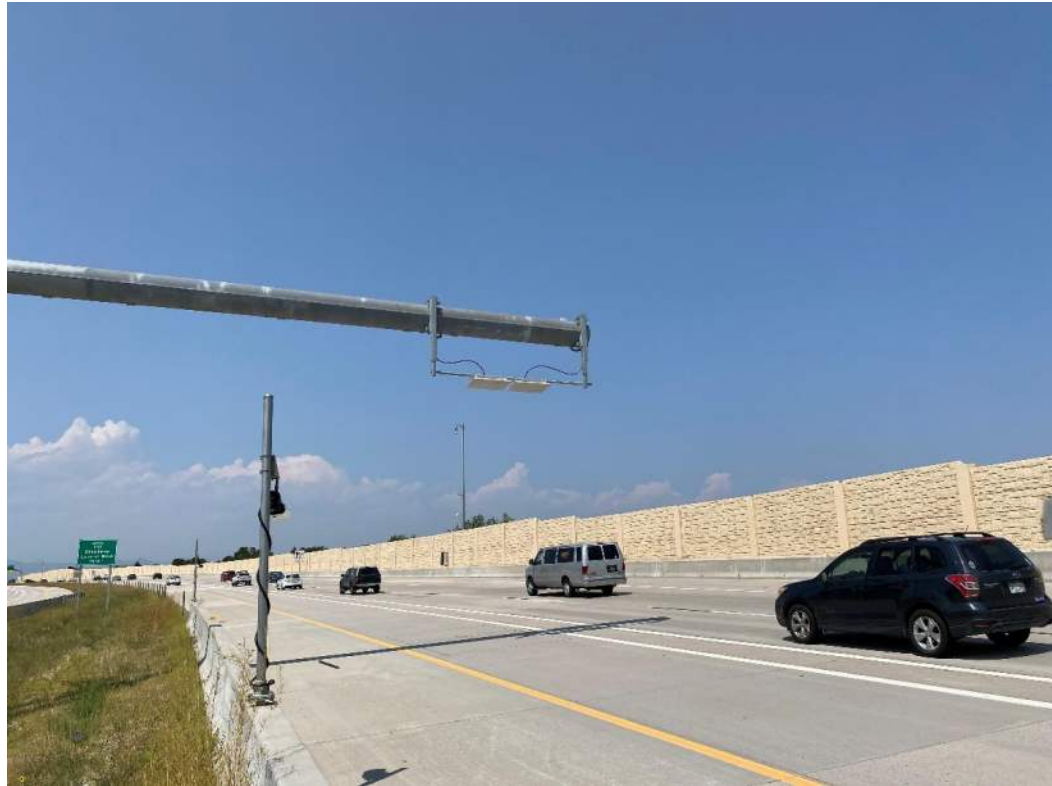
Typical Tolling Device, Good Condition
