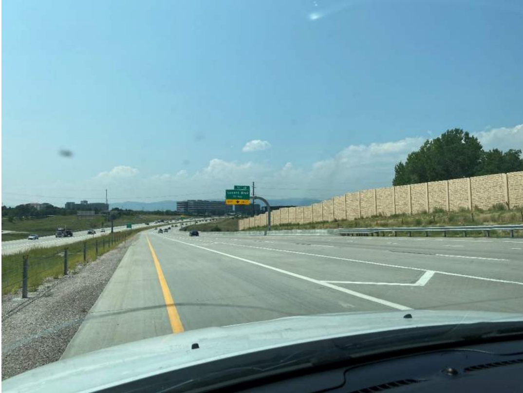
Typical Shouldering and Delineation, Good Condition
