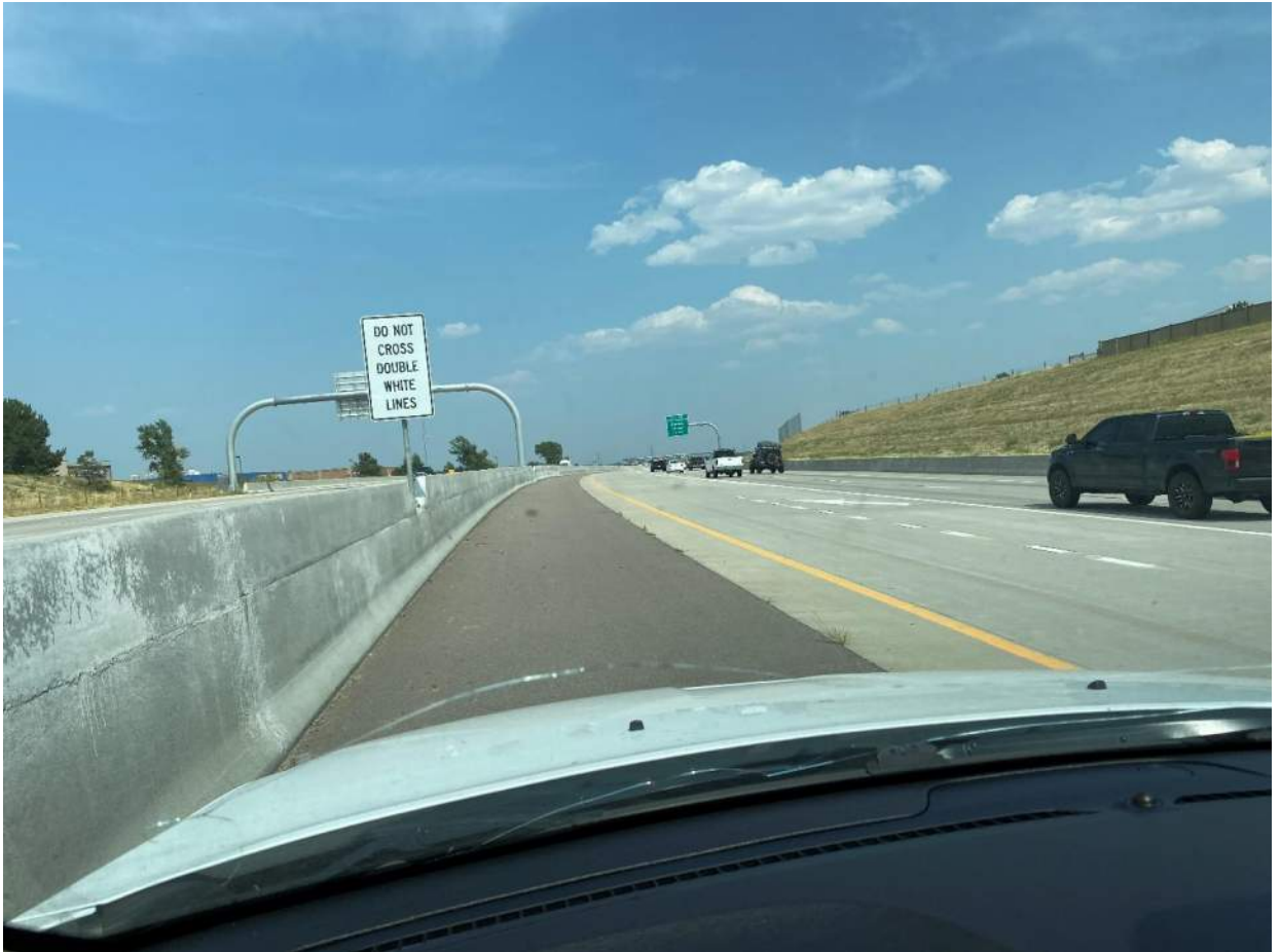
Typical Pavement, Good Condition
