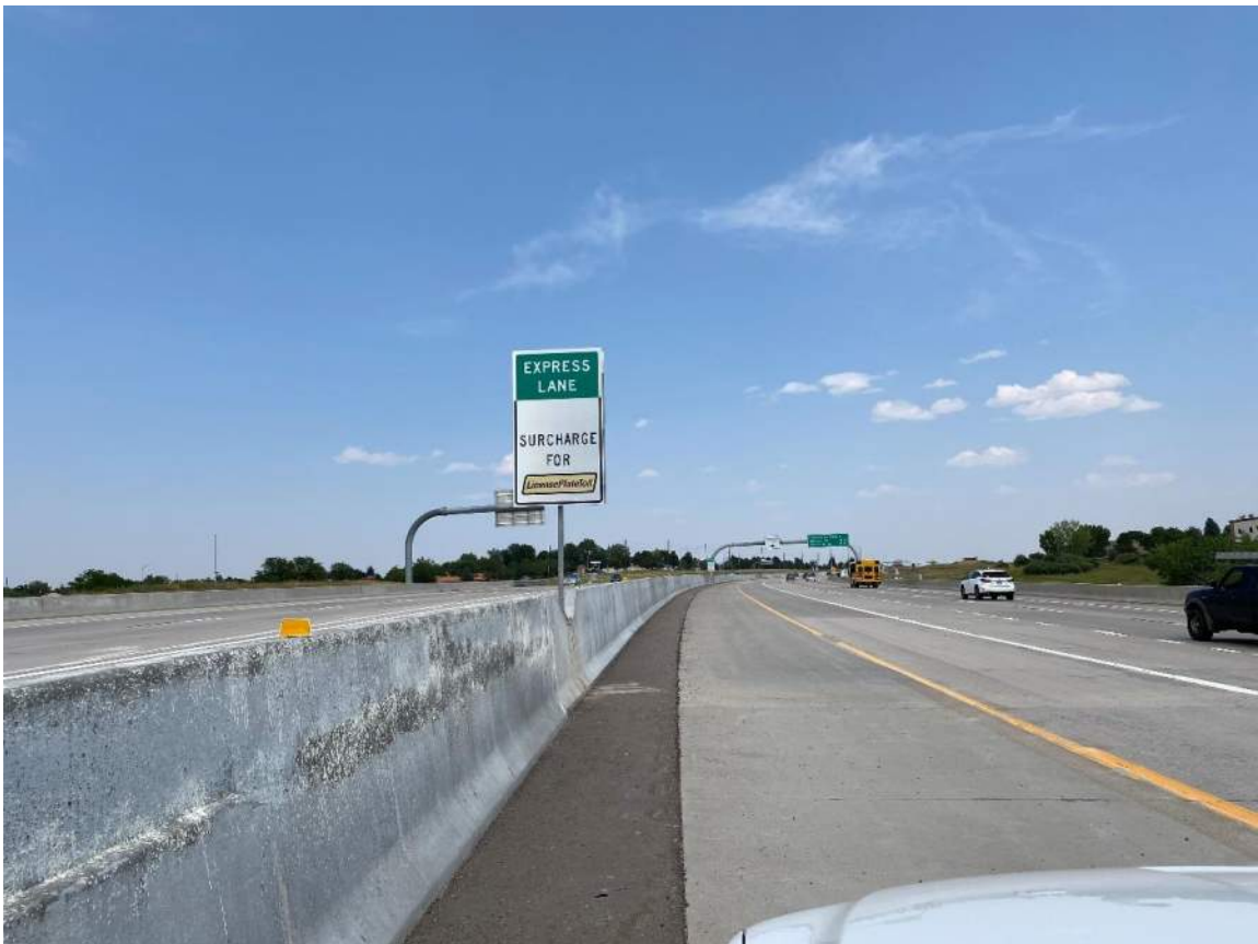
Typical Median Barrier, Good Condition
