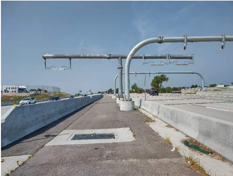
Typical Monotube Overhead Sign, Good Condition
