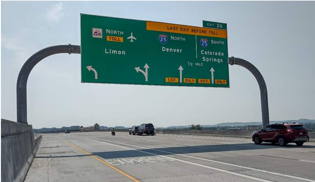
Typical Directional Overhead Sign on Monotube, Good Condition
