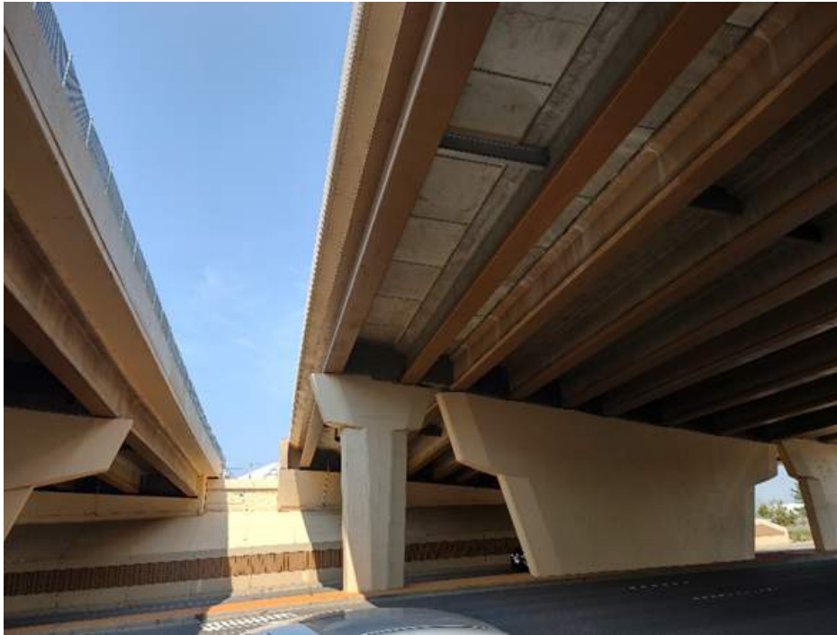
Typical Widening University and Broadway, Good Condition
