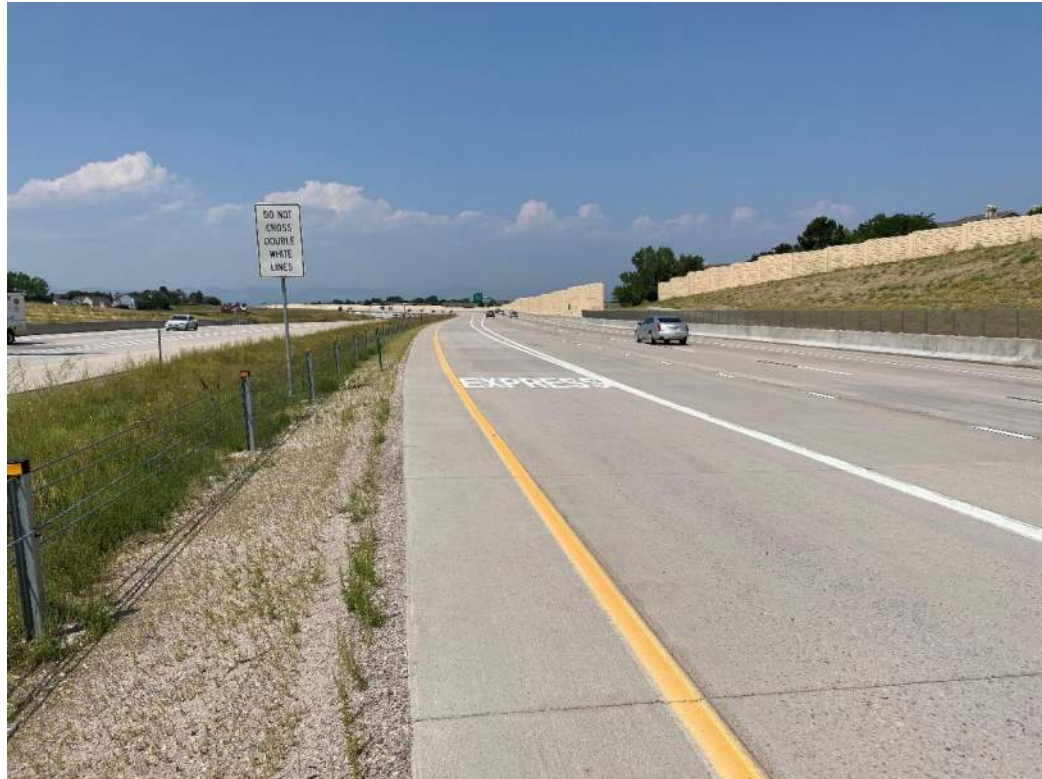
Typical Striping and Lane Marking, Good Condition
