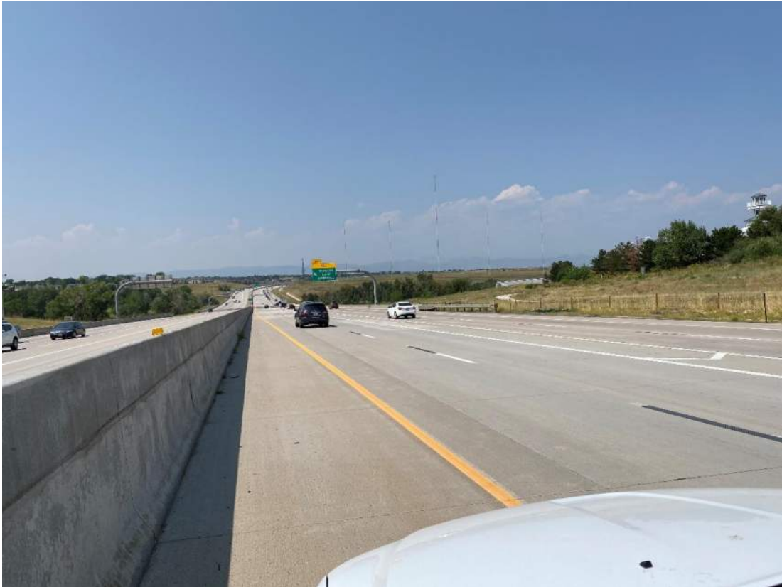
Typical Median, Barrier separated in WB zone 1
