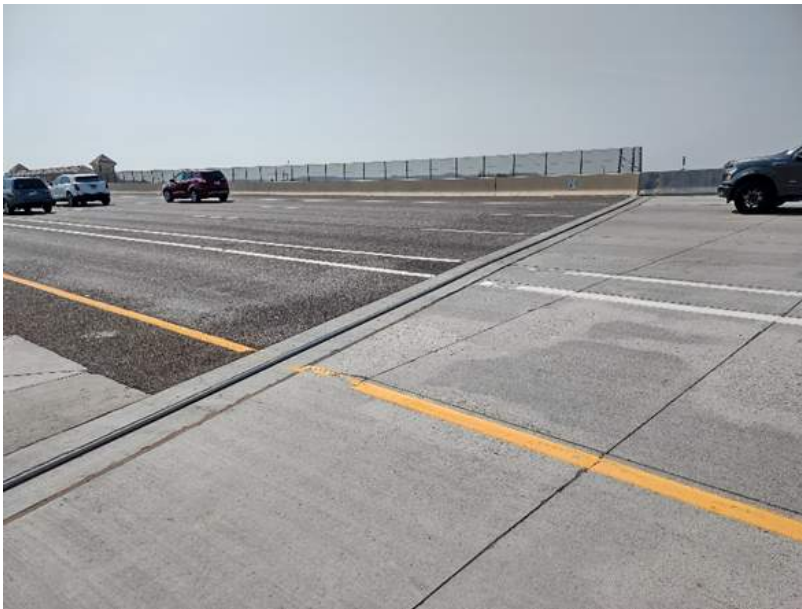
Typical Bridge Expansion Joints, All Good Condition
