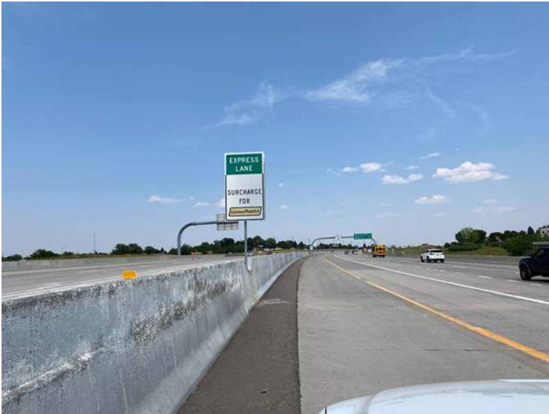
Typical Pavement, Condition Good
