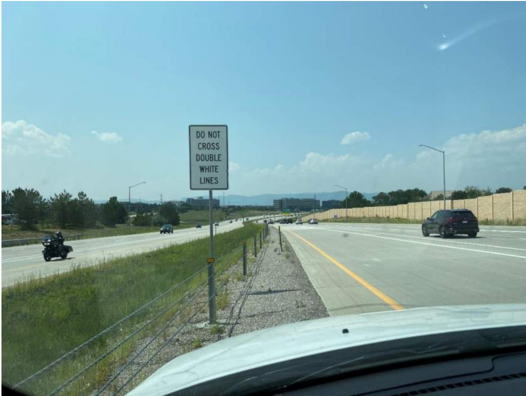
Typical TL4 Barrier, Condition Good
