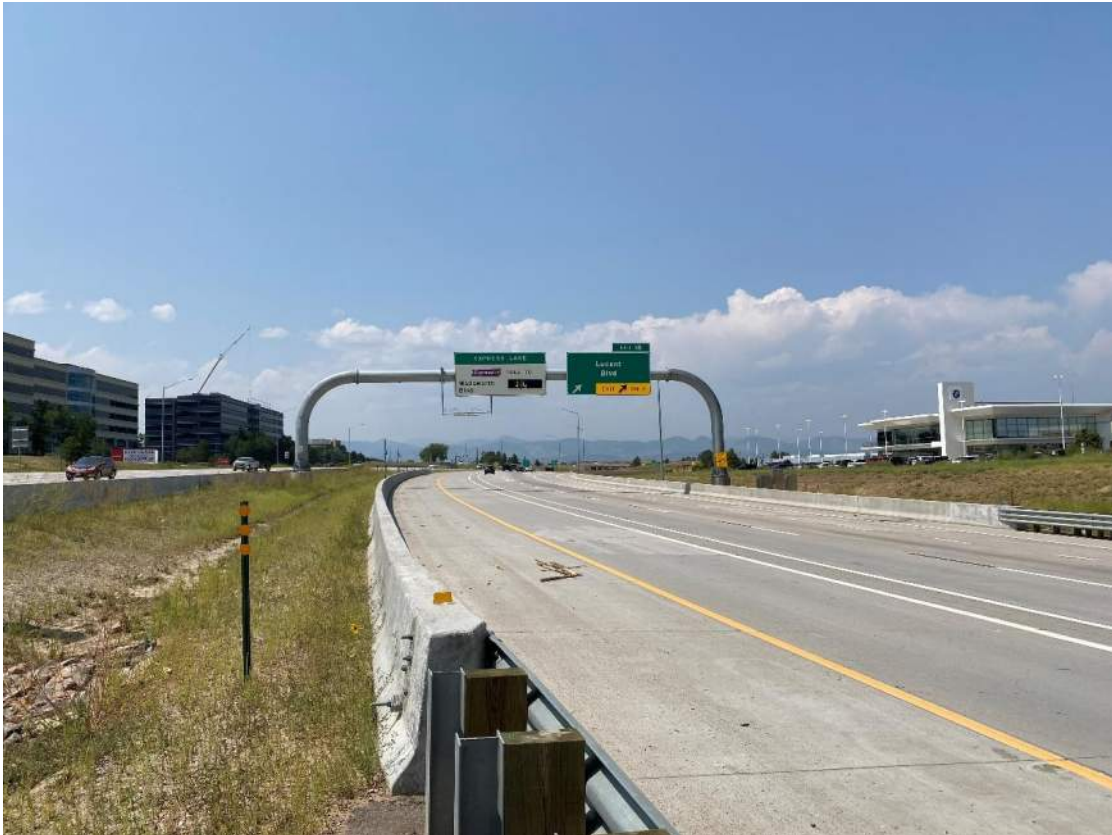
Typical Barrier and Guardrail Transitions, Good Condition
