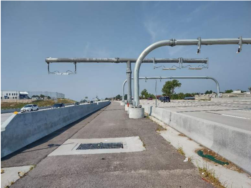
Typical median inlet in good condition
