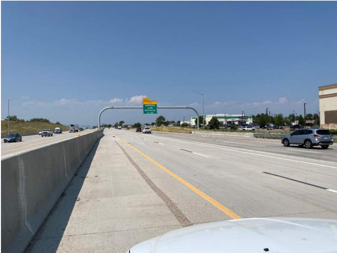
Concrete pavement in good condition. Temporary striping removal evident, no issue.
