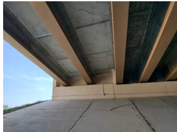
Example, Slope Paving Repair Acres Green
