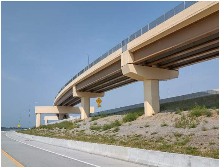
WB E470 to WB C470 Flyover, Good Condition
