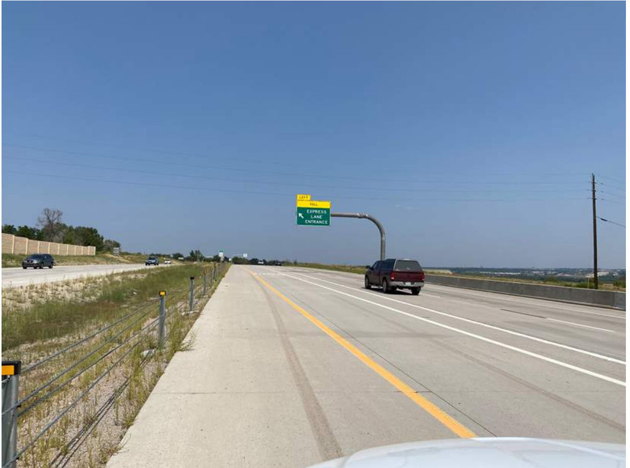
Typical Roadside Shouldering and Delineation, Good Condition
