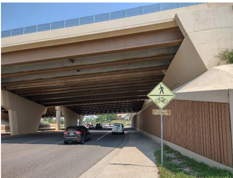
Yosemite Overpass, Good Condition
