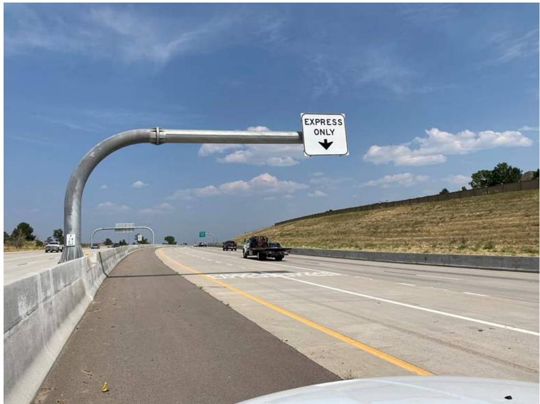
Typical Express Lane Marking, Good Condition
