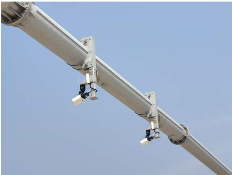
Typical Tolling Device appurtenances, Good Condition
