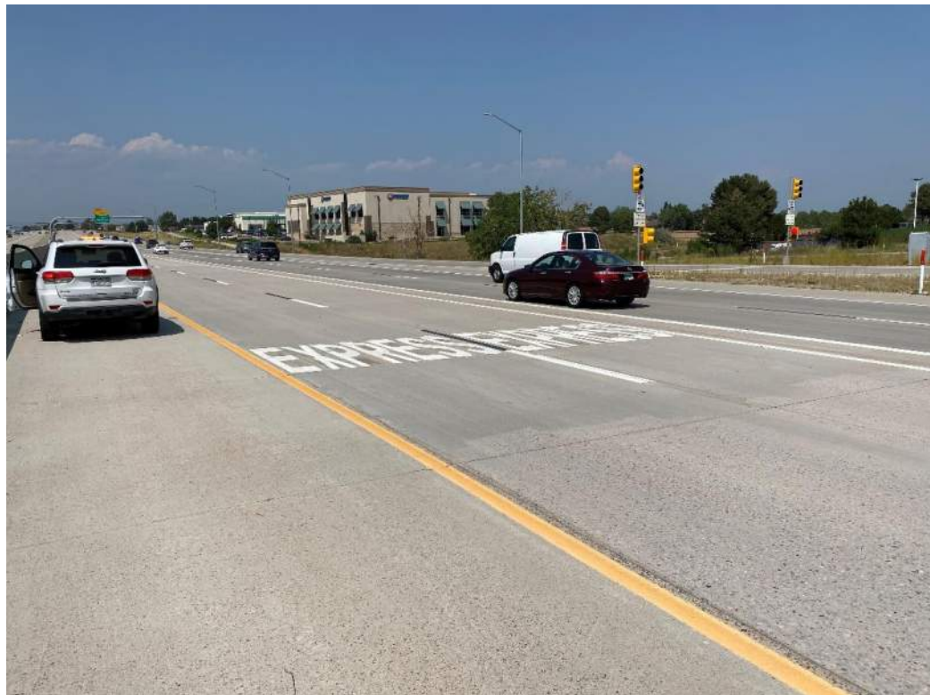
Typical Striping and pavement markings, Good condition.
