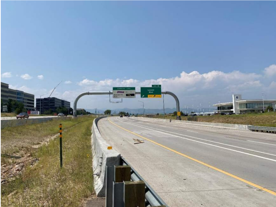
Typical Median, Barrier, and Grading, Good Condition
