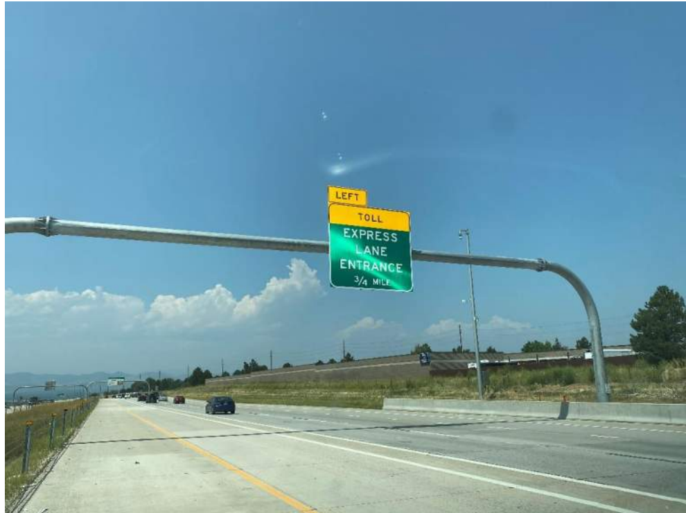
Typical Monotube Overhead Signing, Good Condition
