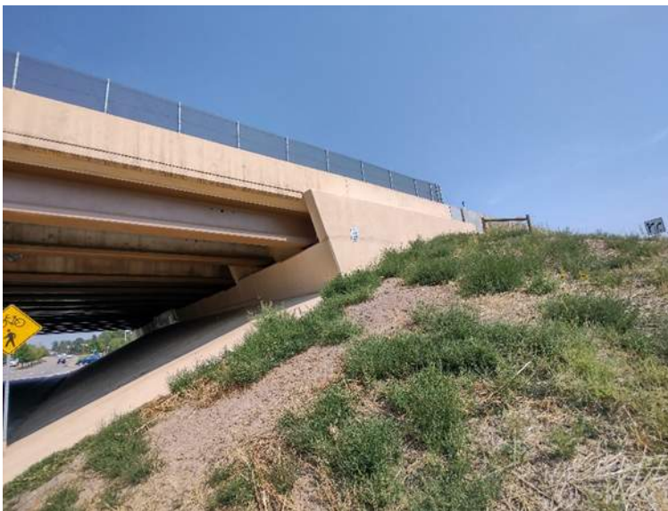
Typical Widening, outside, Broadway and Yosemite
