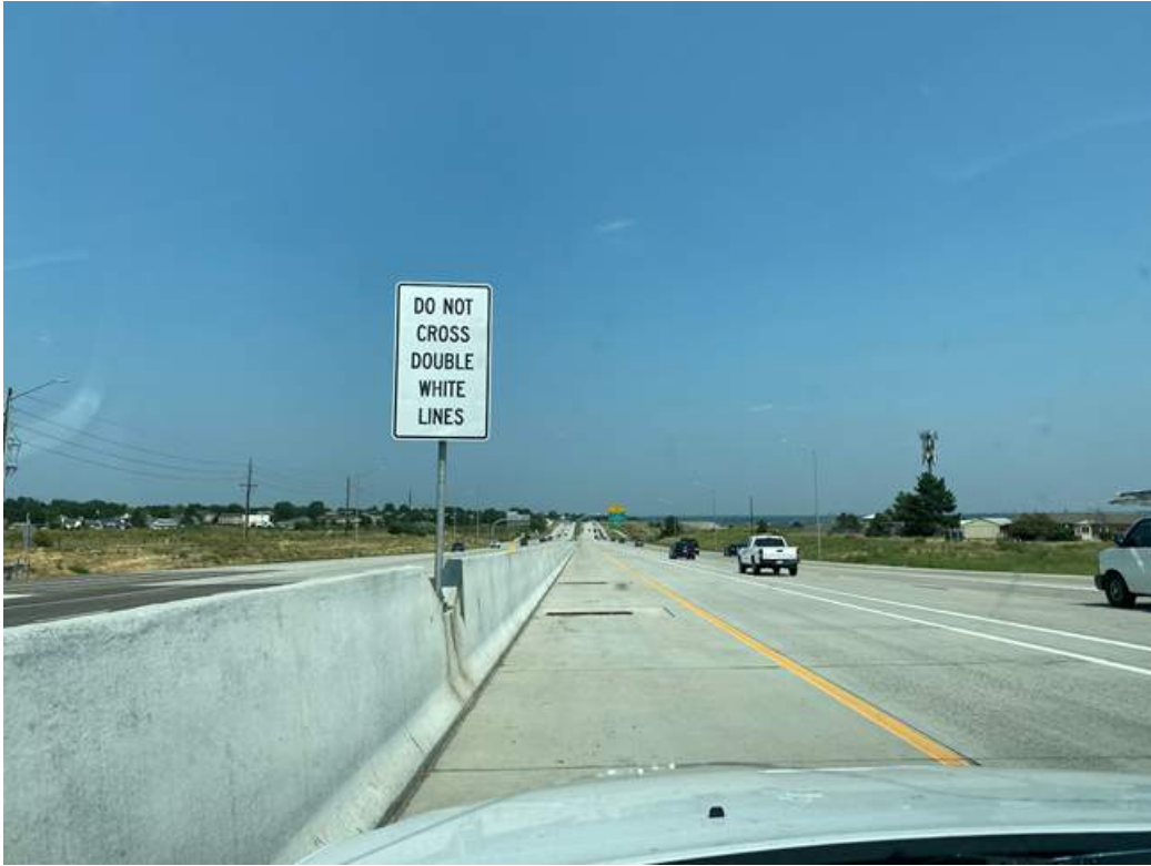
Typical Median Inlets, Good Condition
