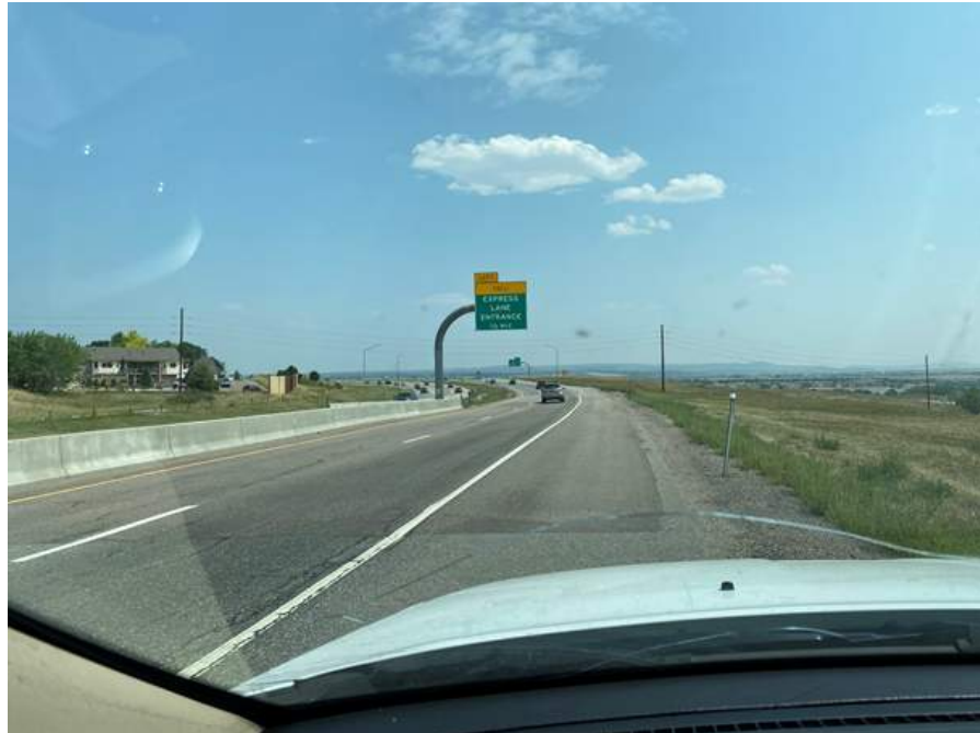
Typical Monotube Overhead Signing, Good Condition
