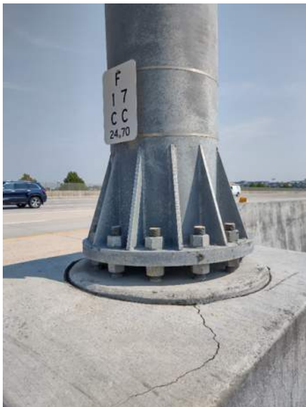
Example, Sign Base Crack Repair
