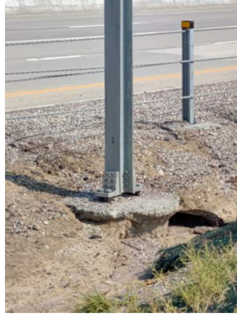
Example, Sign Base Erosion/Repair
