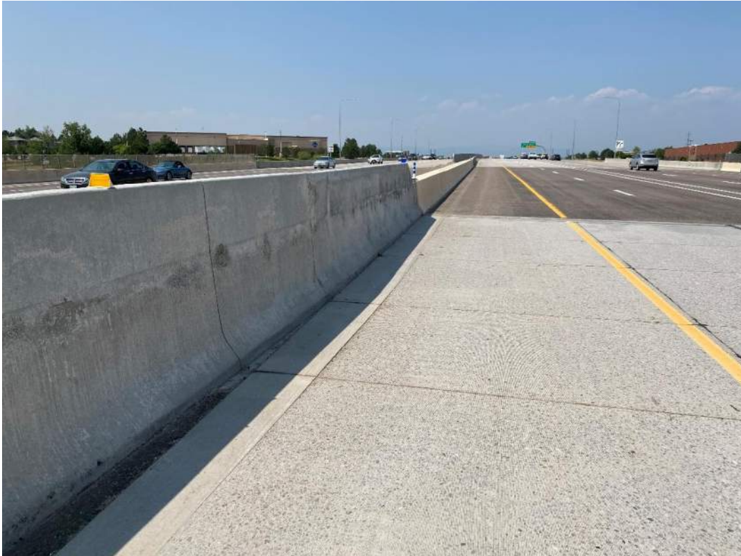
Typical Delineation on Type 7 barrier and bridge rail, Good condition
