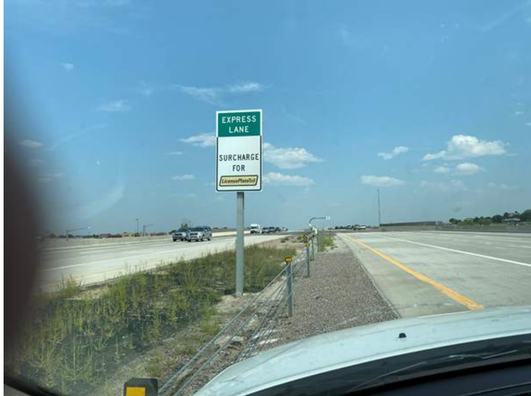
Typical Steel Signpost, Good Condition
